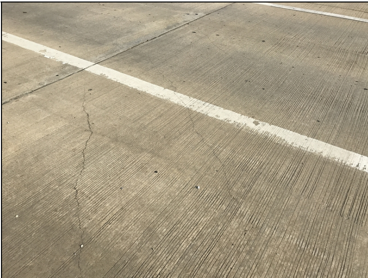
Corner cracks
